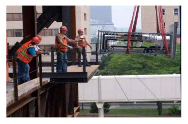
Figure 5. MEP ceiling rack being hoisted to the landing platform with lifting straps (Source: Skanska USA Building)
